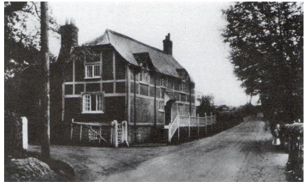
Maintenance Man's House for Upper Lostiford Mill (Demolished 1920s)
